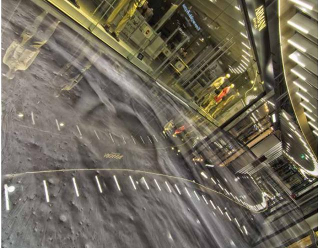
Once mixed, Sikafloor®-160 was put down as a self-leveller at 3 - 4 mm in thickness. As the epoxy flowed and the 40-minute curing process began the shards settled and created the desired metallic cloud patterns with a translucent 3D effect.
