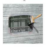
Step 4: Application of Bonding Agent Sikadur® 32 LP/ Sika®-Hibond/ SikaTop®-Armatec-110 EpoCem®
