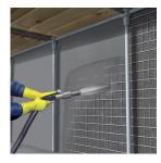
Step 2: Rust Removal of bars using Sika® Rustoff 100
