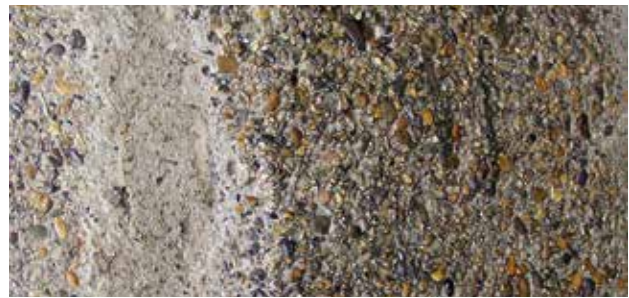
Due to continuous exposure, the cement film is eroded in an initial step, and thereafter larger and larger aggregates are rubbed, knocked or washed out of the hardened cement paste
