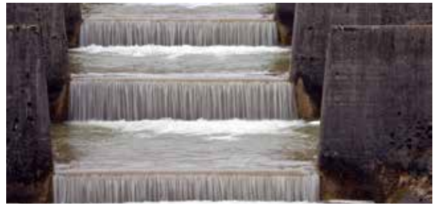
Particularly in whitewater, concrete surfaces are subject to massive additional strains by rubble, sharp edges and abrasion, as well as possible temperature stresses due to frost exposure.
