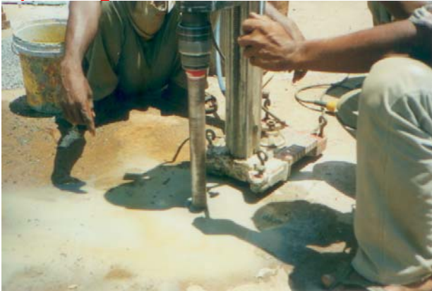
Holes to fill in micro-concrete from the topside
