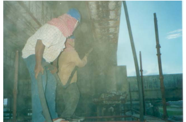
Sandblasting operation in progress.
