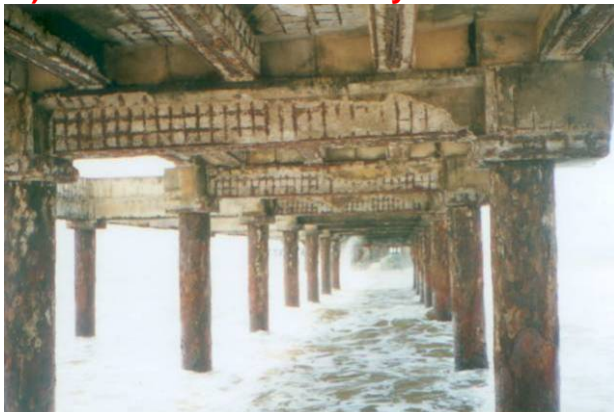
Full view of underside of Jetty
