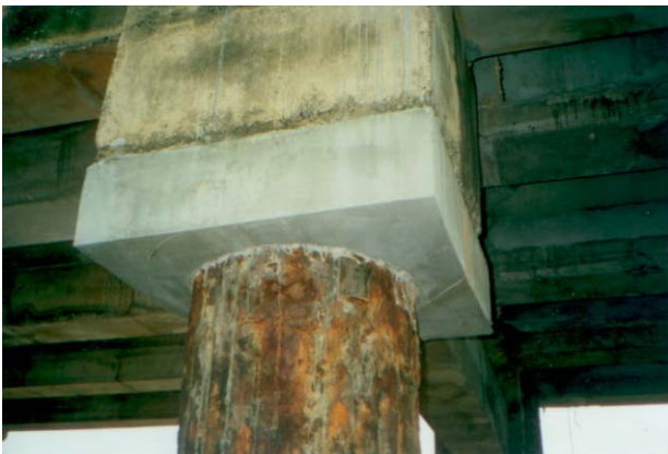
Detail refurbished pile cap
