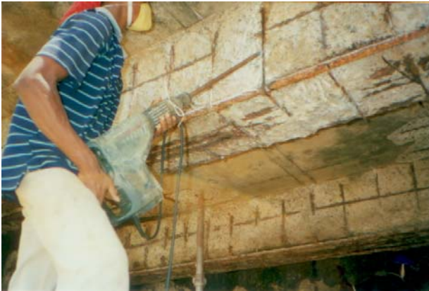
... and a power driven chisel hammer.
