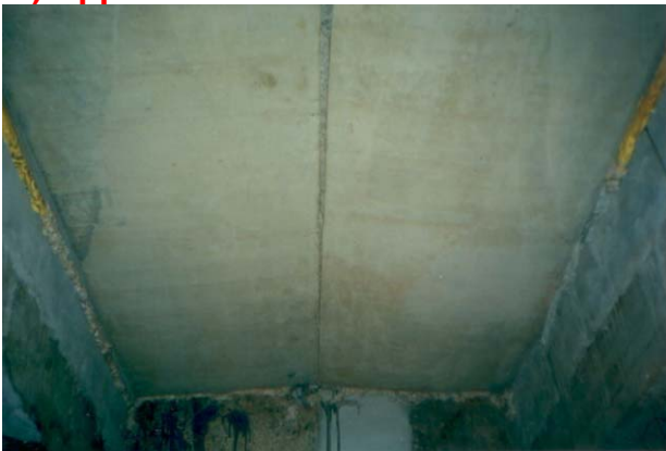
Detail refurbished slab
