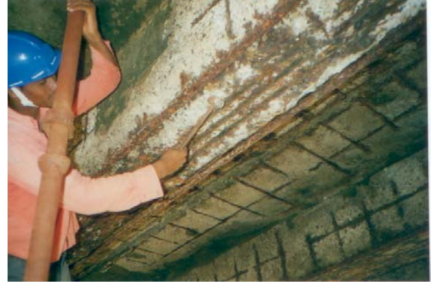
Removal of loose concrete using a chisel ...
