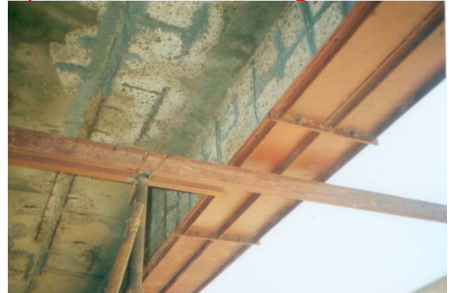
Part-shuttering for the beam installed
