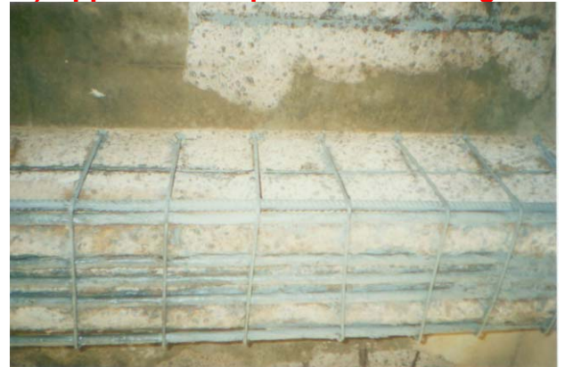
Protective coating applied on rebars
