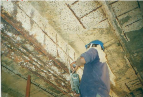
Drilling of holes to fix additional stirrups
