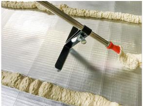
Apply the appropriate amount of SikaRoof<sup>®</sup> Board Adhesive according to the roof wind-load zone requirements.
