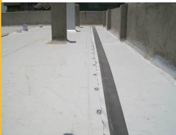
Spot-fixed membrane overlap prior to welding of membrane cover.
