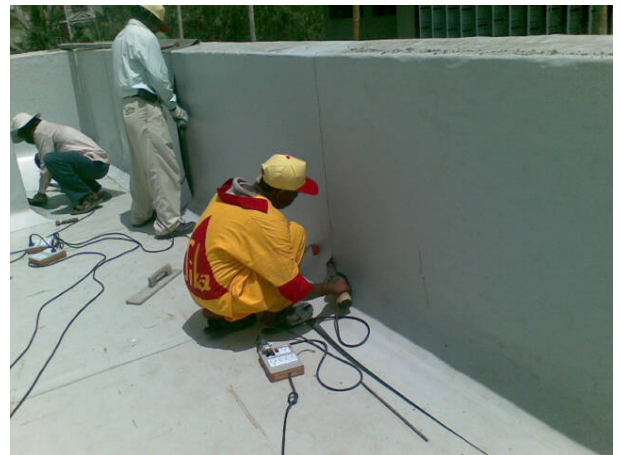
Welding of the PVC membrane overlaps.
