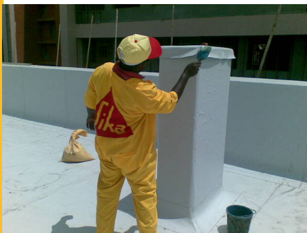
Installation of column cover flap.
