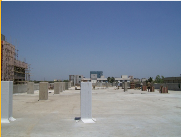
Cleaned concrete substrate.
