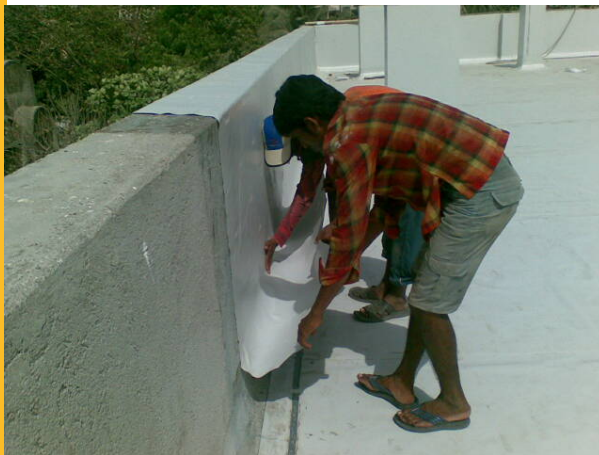
Placement of the up stand PVC membrane.
