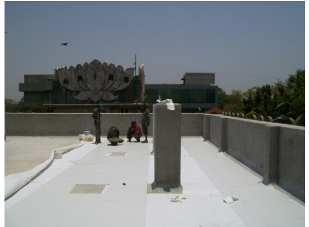
Pre-cutting of PVC membrane on top of geo textile.
