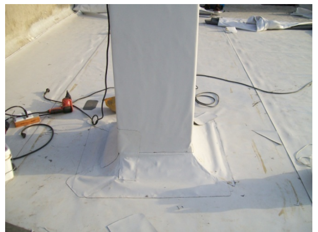
Finished roof column detail.
