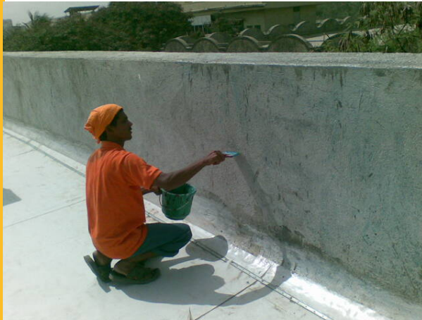
Application of the adhesive to the up stand.
