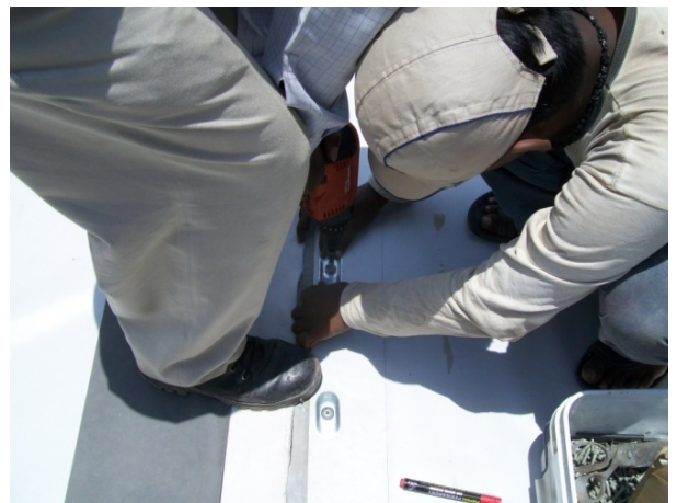
Installation of fasteners along membrane overlap.
