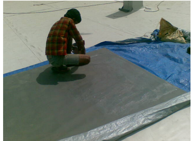
Application of the adhesive to the up stand PVC membrane.
