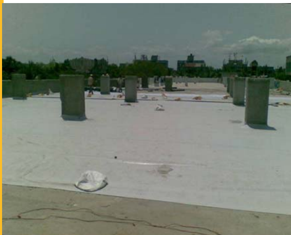
Loosely laid PVC membrane.
