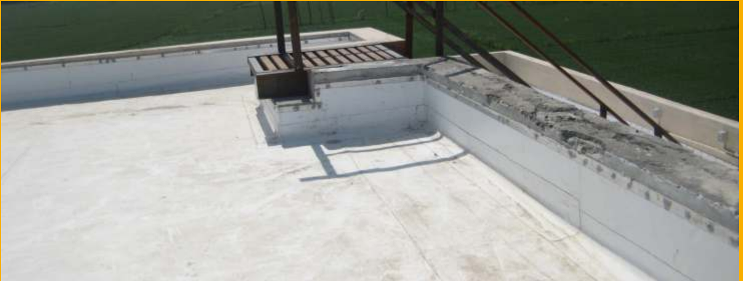
ROOFING WITH SARNAFIL® MEMBRANES AT BAYER CROPSOURCE R&D CENTER, KARNAL
