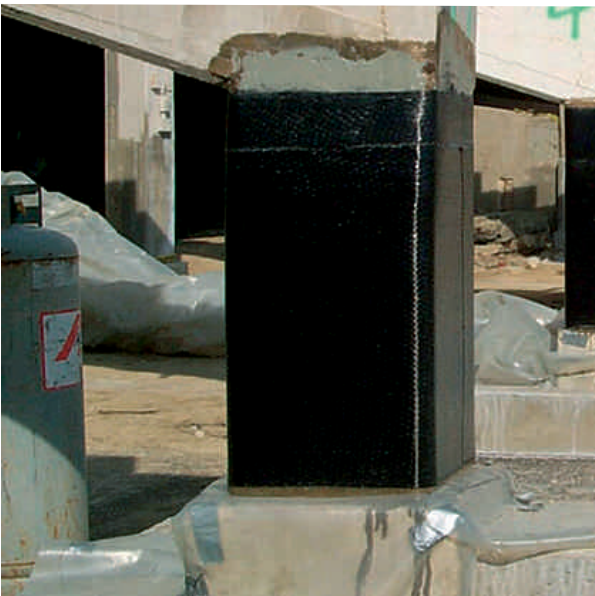
Columns Strengthening (Confinement)
